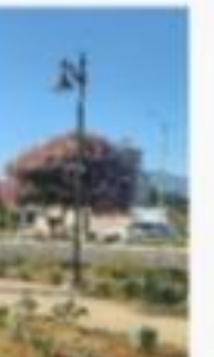
PEDESTRIAN PATH AND PARKING LOT LIGHT
